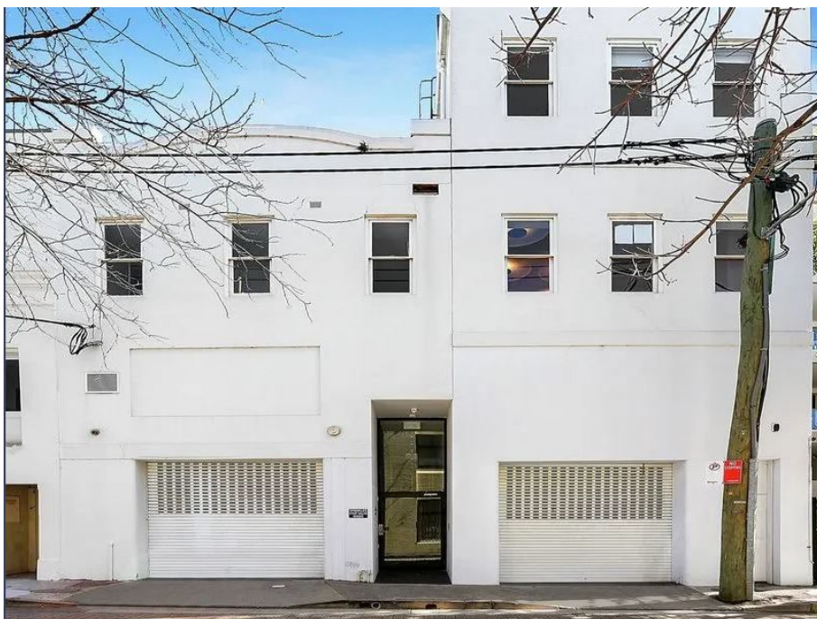
21 Rear elevation of 40-42 Flinders Street, on Chisholm Street.
